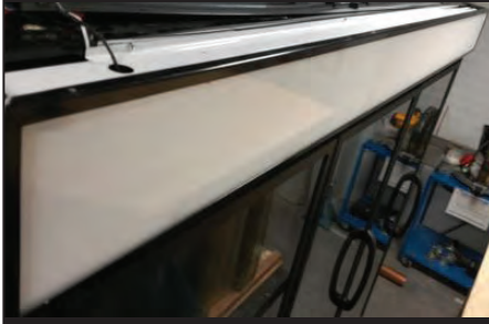
Display Slides out to access Wireway
