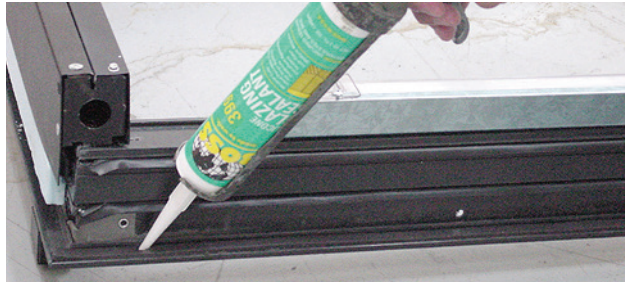
Apply Silicone Sealant
