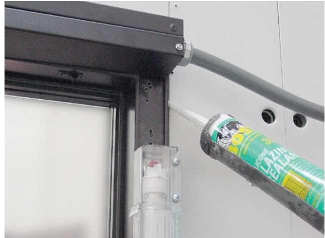
Apply Silicone Around Frame
