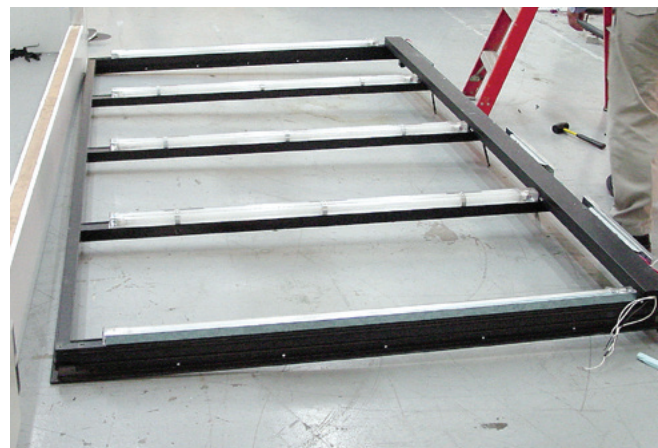
Unpack Frame and Lay Face Down
