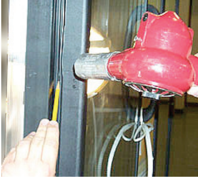
Pulling Gasket Into Place With a Pencil
