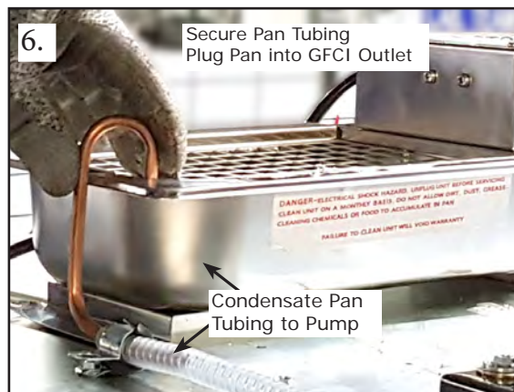
Condensate Pan (Installed on top of case)
