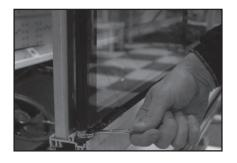
11. Insert wiper retainer at an angle into bottom extrusion as shown in Step #1
