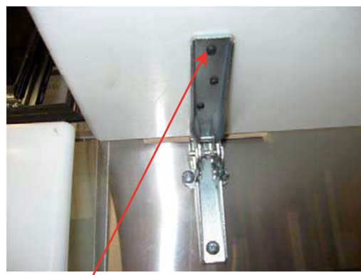
Step 8: Screw bracket into wrap board (screws provided #8 X 1 1/4")
