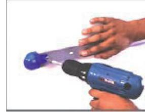
1. Attach the base and end/corner cap to the desired surface by inserting #8 pan head screws through the pre-slotted holes in both the end cap and the base. Insert screws through the two holes of end cap and tighten.
